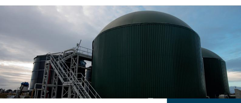
EPS builds and operates anaerobic digestion systems in Ireland at multiple municipal wastewater sites. Anaerobic digestion (AD) technology allows for the generation of renewable energy from the sludge treatment process.
