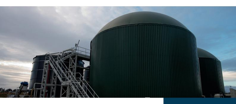
EPS builds and operates anaerobic digestion systems in Ireland at multiple municipal wastewater sites. Anaerobic digestion (AD) technology allows for the generation of renewable energy from the sludge treatment process.
