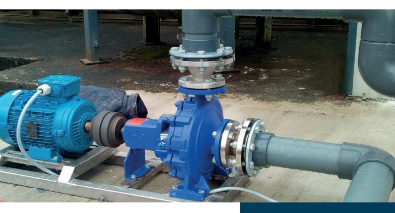
EPS supported the installation, maintenance and monitoring of a micro-hydropower energy recovery system at the EPS operated Blackstairs Group Water Scheme site in Co. Wexford.
