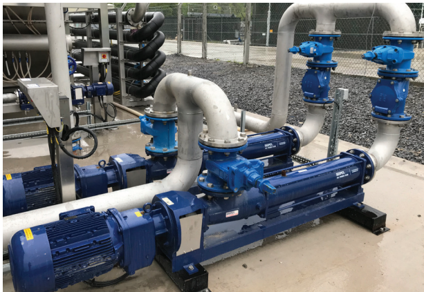
➤ Progressive Cavity Pumps
