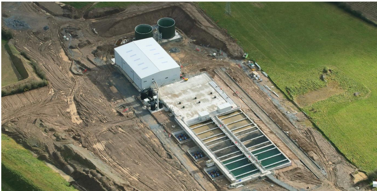
Photo 1: New Wastewater Treatment Plant under Construction (Jan 2017)
