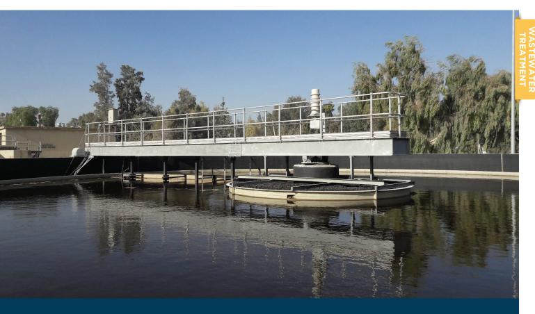
The overall project entailed the upgrade of the two wastewater treatment plants at Central Irbid (250,000 PE) and Wadi Arab (140,000 PE), to achieve wastewater suitable for agricultural re-use after nitrogen removal, filtration and disinfection. EPS entered into a joint venture with local civil partner, El Concorde Construction and were successful in securing the contract.
